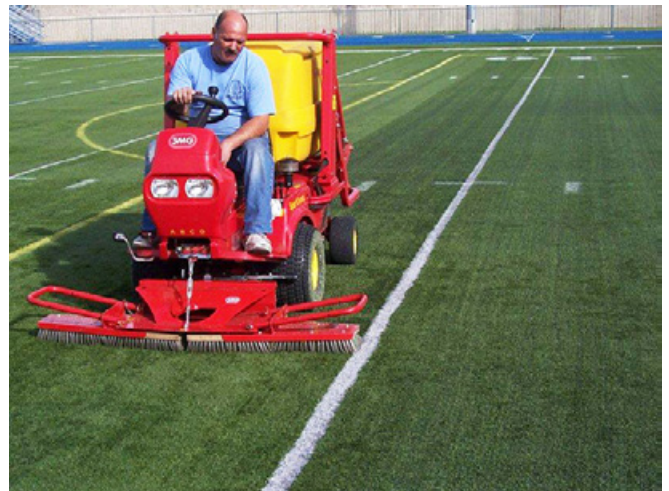
Figure 1 - brushing of a synthetic turf surface to help redistribute any dispersed infill.
