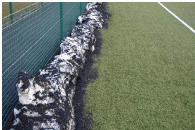
Figure 2 - snow being stored on the side of a synthetic turf field to ensure infill does not contaminate the surrounding environment.
